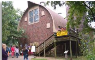
Indian Creek Nature Center's Old Barn
